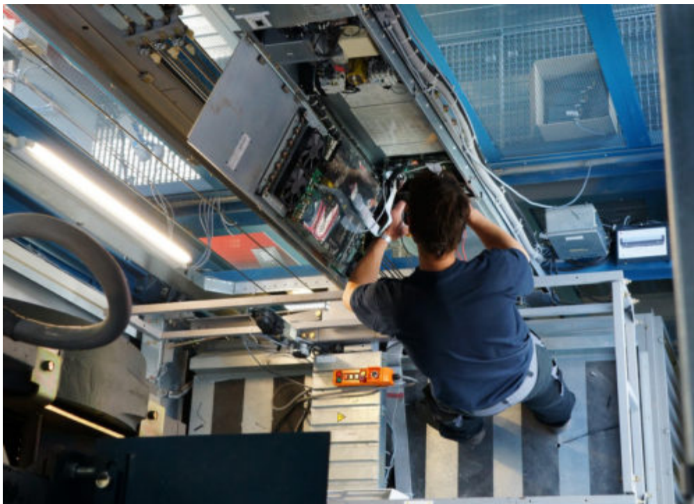
FIGURE 13 MAINTENANCE OF MITSUBISHI ELEVATOR
