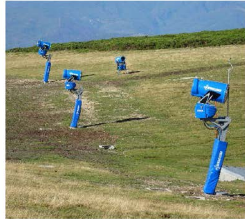
Figure 8. Snow cannons installed in 2018 and 2019. Source: Photo from the authors' files (16/08/2019).
