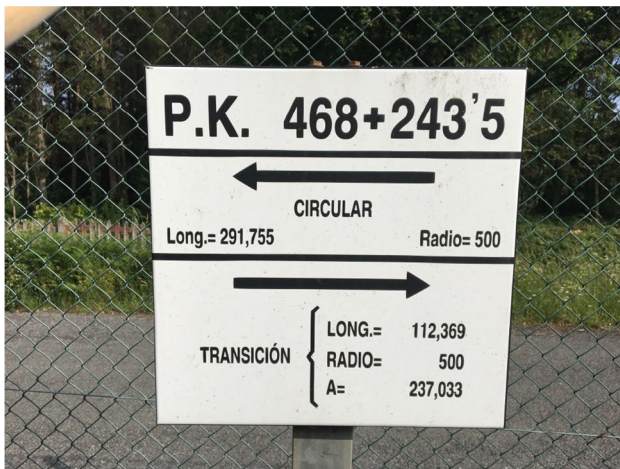
Fig. 6 Informative board located along the railway track with geometrical information about the horizontal alignment elements
