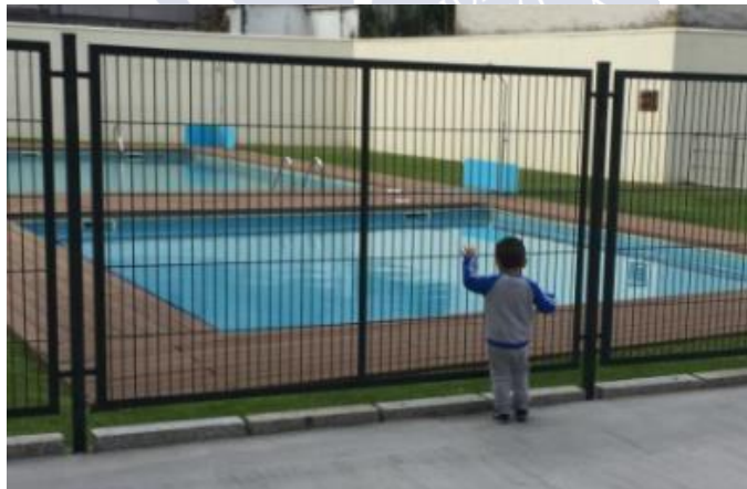
Figure 2. Prevention mechanism. Perimeter fence preventing free access to the pool (own photograph).
