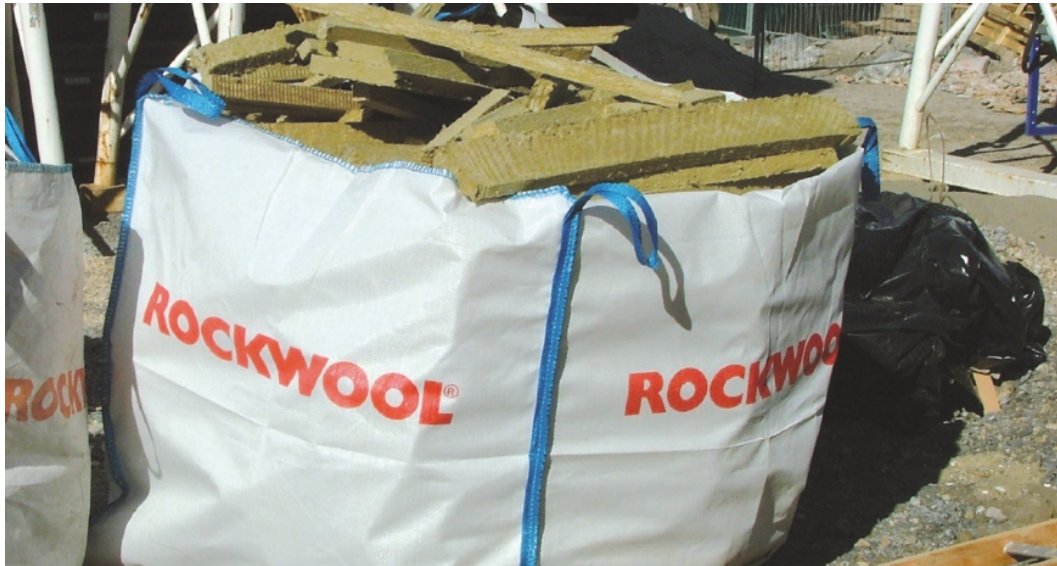
FIGURE 12: TAKE BACK OF EXCESS MATERIAL
