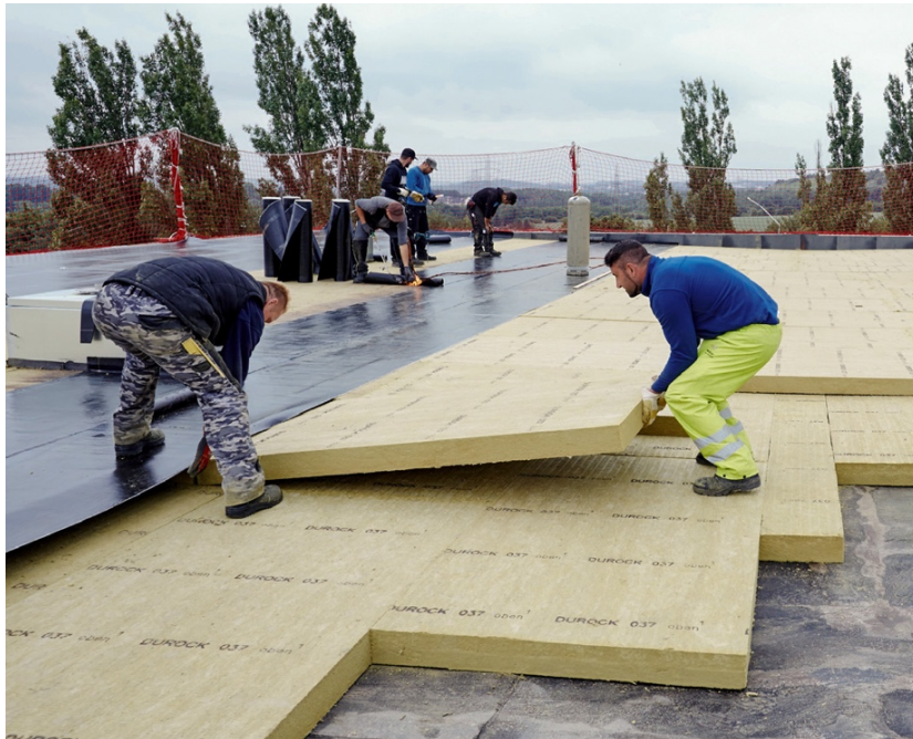
FIGURE 13: FLAT ROOF INSULATION
