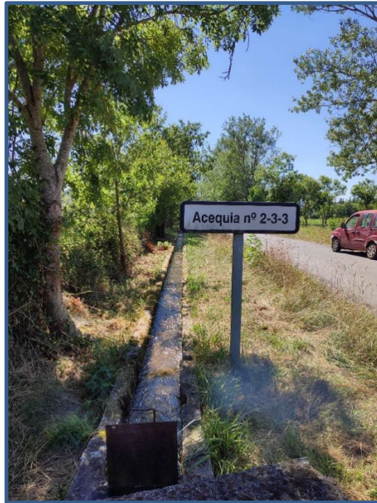
Image 4.2.2.16. Secondary water distribution channel
