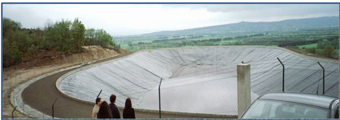
Image 4.2.2.7. Water storage pond in the 'A Limia' region. Irrigation modernization actions
