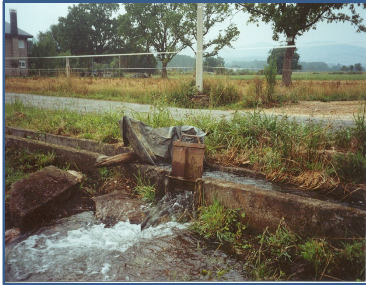
Image 4.2.2.8. Example of the misuse of water in the Lemos Valley irrigation area, with low efficiency
