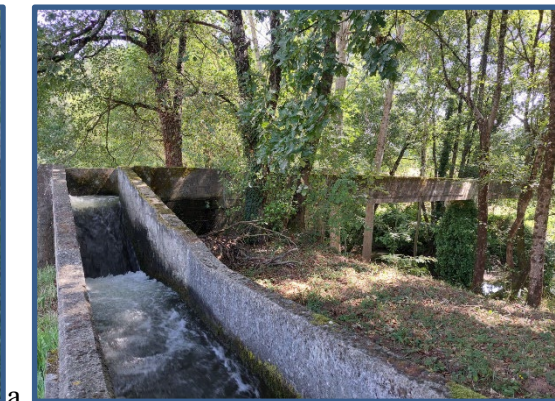
Image 4.2.2.15. Infrastructures for passage of topographic obstacles in Lemos Valley: a) siphon and b) aqueduct
