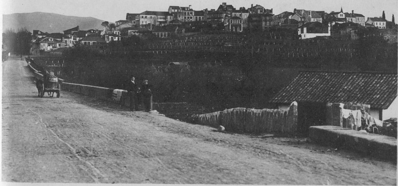
PUENTEAREAS — Vista general
