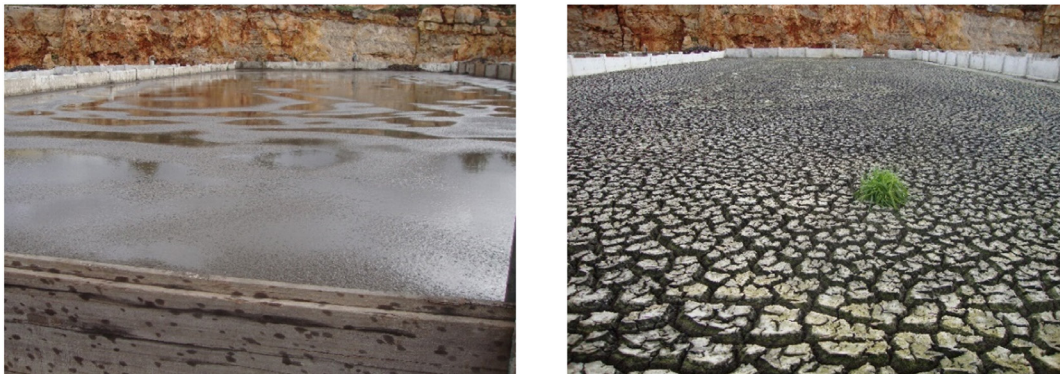
Figure 6.13 Sludge-drying bed in a municipal STP containing fresh sludge (left) and with dehydrated sludge (right).
