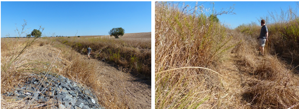
Figure 53. Practical activities in EDIA: drainage system maintenance.
