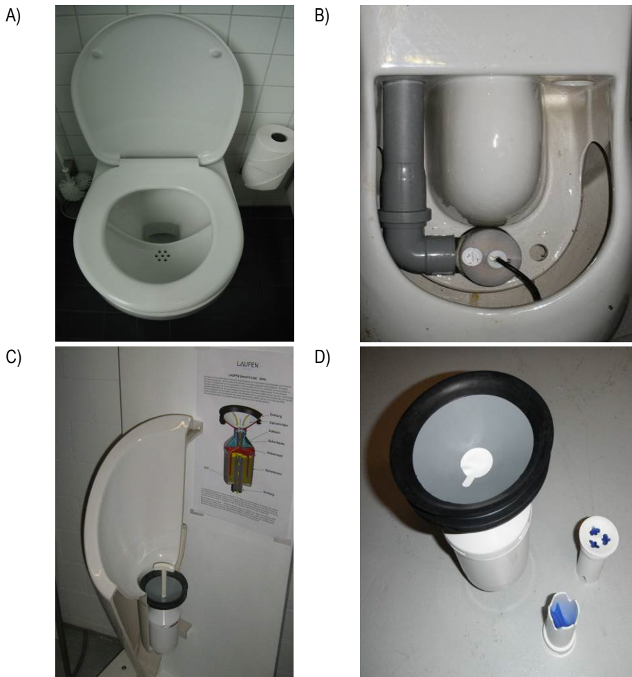
Figure 5.1. A) No-Mix toilet. B) Bottom side of a Roediger NoMix toilet. When somebody sits down on the toilet the valve is opened and the urine can flow out through the grey pipe into the urine collection tank. C) Section view of a water free urinal. D) Siphon and membranes of a water free urinal.
