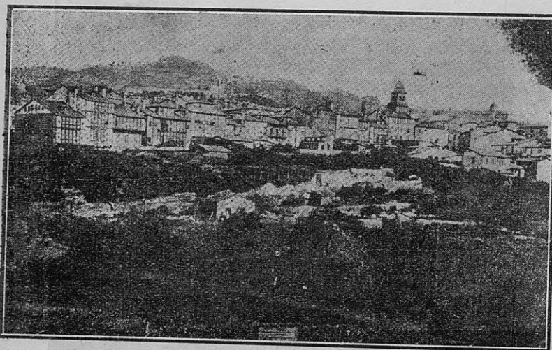
ORENSE. — Vista General
