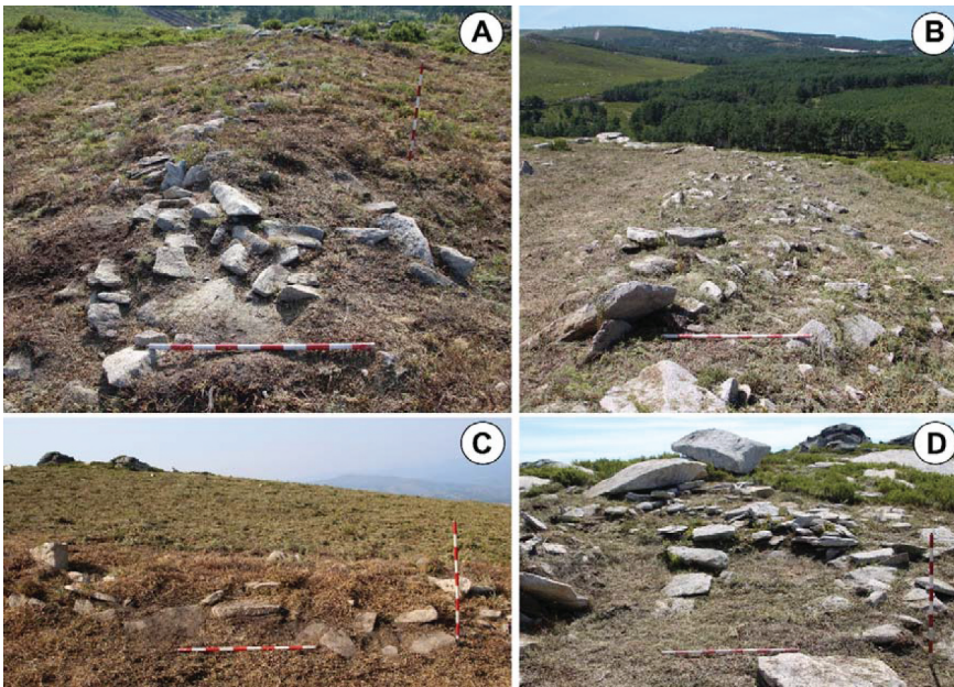
Figure 7. Front and rear revetments as seen in the southern (A, UE001) and northern (B, UE012) ramparts; front revetment of the rampart laying over an earthbank (C, UE002); and northern clavicula entrance (D, UE011 and 012).
