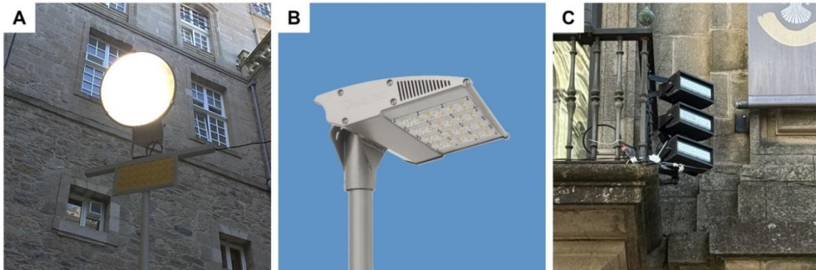
Figure 34. Photographs of the three ornamental lighting systems considered in the current study. A) Metal halide system (image provided by P. Sanmartín), B) white LED system (image provided by Televés S.A.U.) and C) CromaLux system (image provided by A. Méndez).
