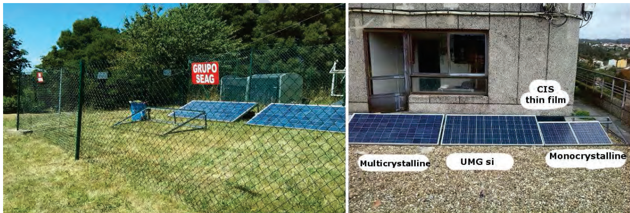
Fig. 57 Monitored photovoltaic installations in Santiago de Compostela, near to a MeteoGalicia [188] weather station.
