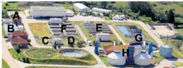
Figure 1 | Aerial photograph of the wastewater treatment plant Grevesmühlen.
