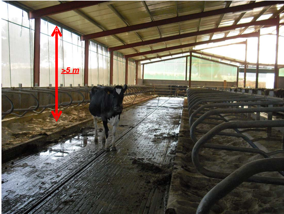
Picture 8.- Promoting natural ventilation will help to maintain a healthy environment. Open sides ensure air circulation through the barn
