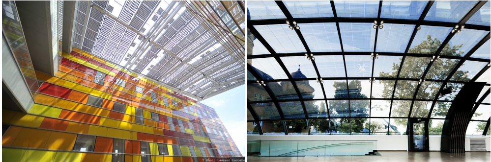
Figure 1.4: Two examples of BIPV (left c-Si [14], right a-Si:H [15] technology).
